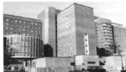
Blending in evenly with the brick exterior of the Clinical Center is the one-story In Vivo NMR Research Center, adjacent to the CC's D wing.
